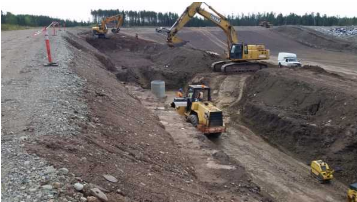
Photo – 2016 Infrastructure Work – Installation of Trunk Lines
