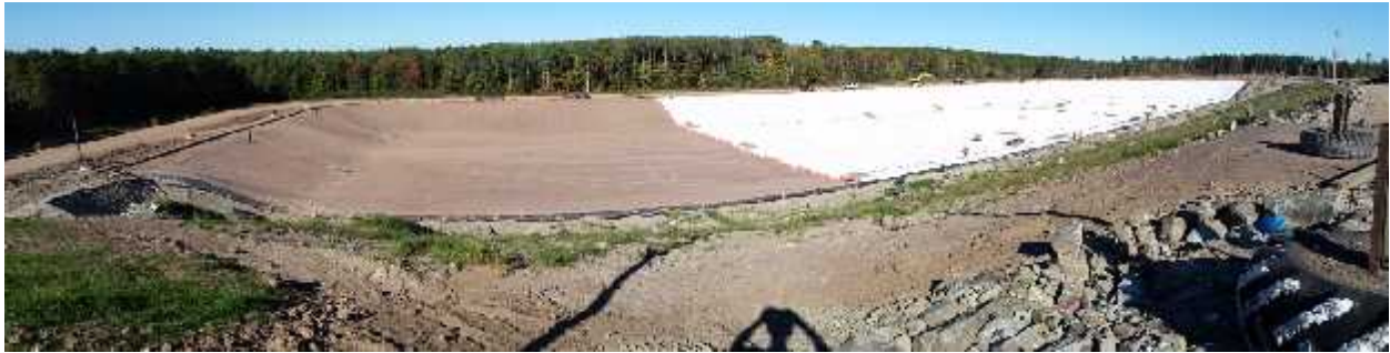
Photo – 2016 Infrastructure Work – Cell # 13
