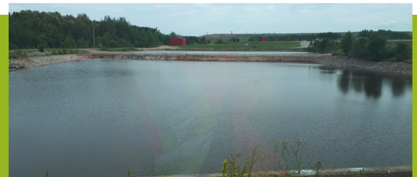
Photo - Sedimentation Ponds
